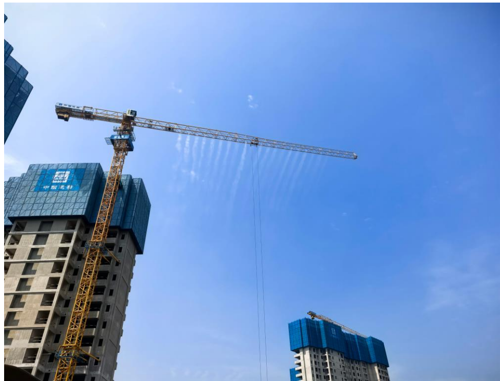
塔吊设置喷淋
